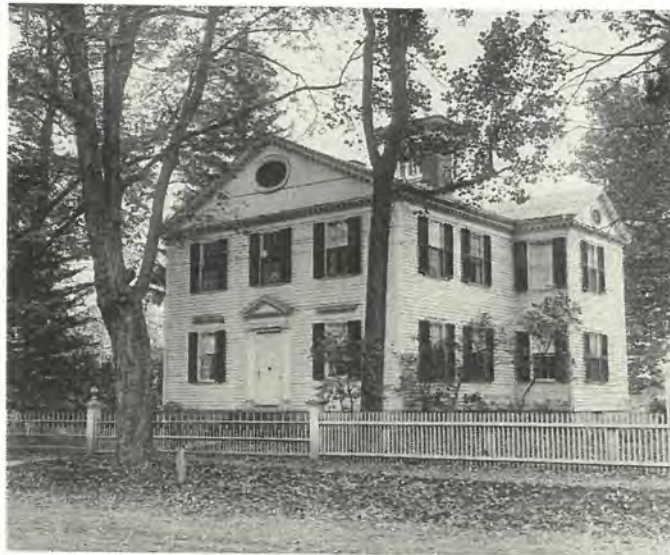
115 Palisado Avenue (Rt. 159). WHS Collections
