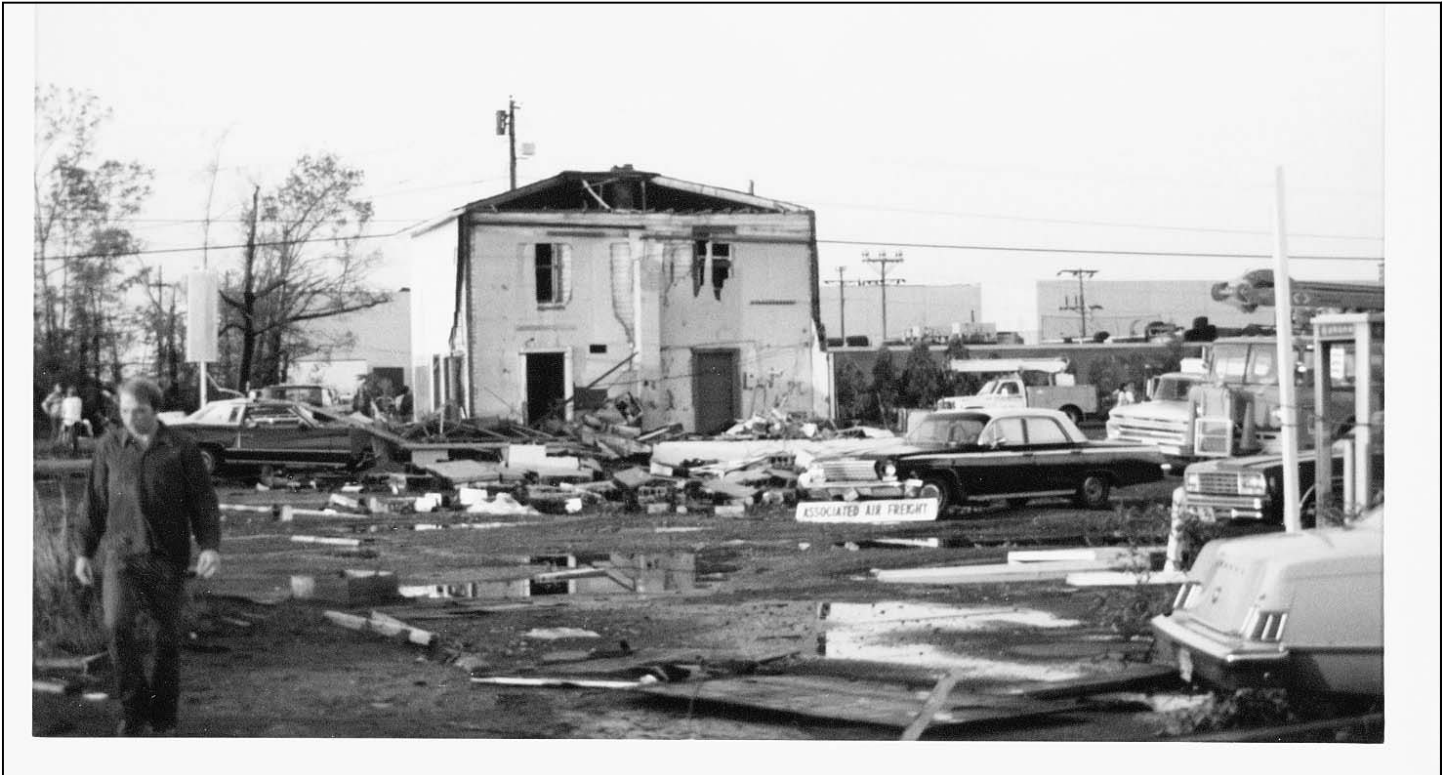
1979 tornado damage. WHS Collections
