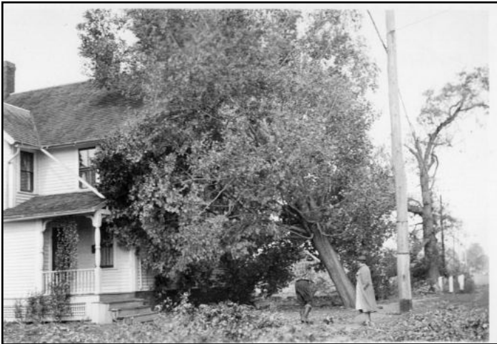
Damage left by 1938 Hurricane. WHS Collections.
