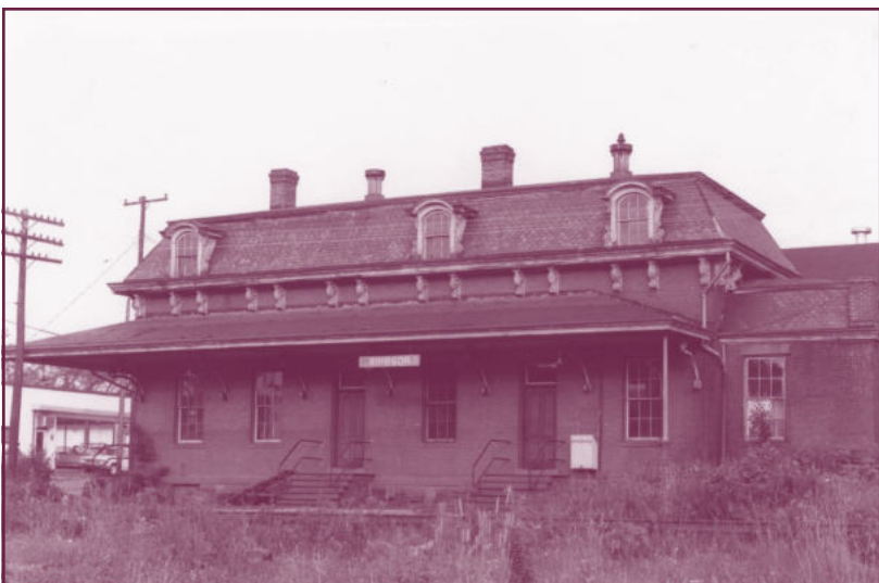
Windsor Train Station in disrepair, 1957. Photo courtesy of Julius Rusavage, WHS Collections.
