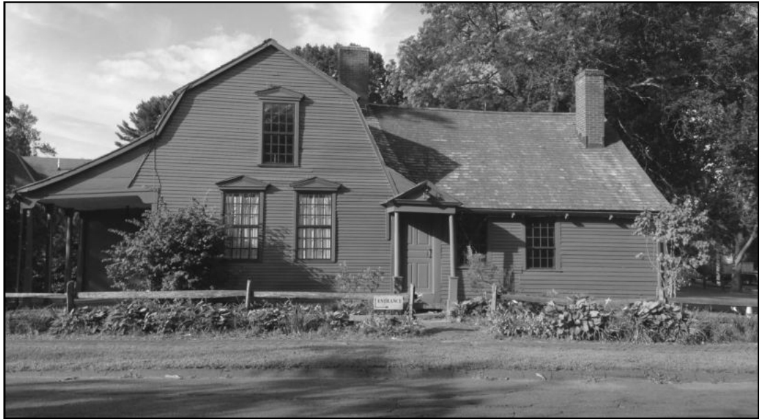
Restored North façade of the Strong Howard House, August 2013
