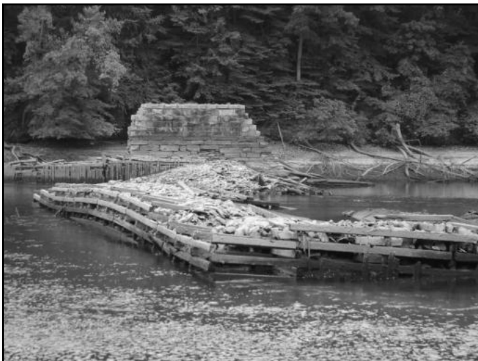
Photo 6: Abutment Remains, 2009 Photography by author, 2010.58.31
