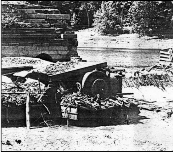
Photo 1: Oil City Dam and Power House Remains, 1976 Richard Daley Photography, Inc., 2010.58.28
