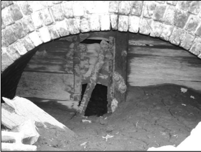
Photo 3: Sliding Input Gate Remains, 2010 Photograph by the author, 2010.58.32
