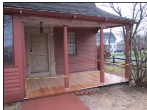
Figure 2: The porch decking has been replaced with long-lasting materials.
