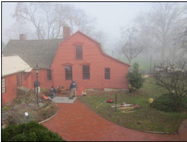
Figure 1: Ironwood Landscaping begins work on the Courtyard drainage, November 23, 2012.
