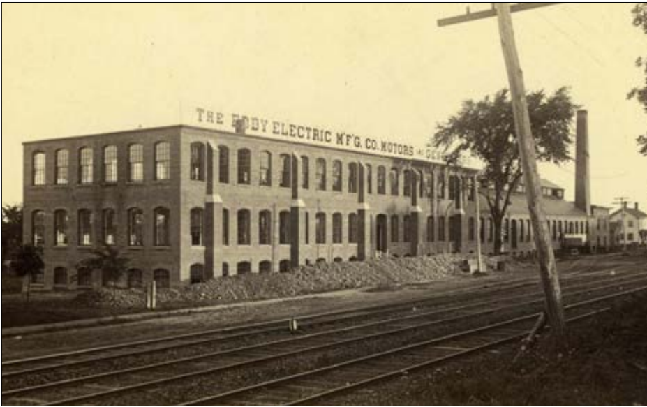
Eddy Electric Manufacturing Company building at 33 Mechanic St. in Windsor, 1892. | WHS collections 2007.1.37, photo by Fred Barry
