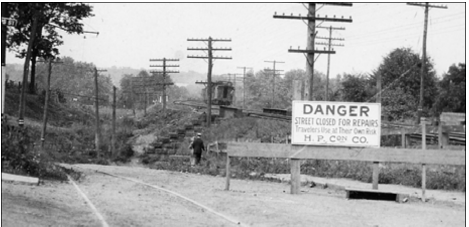
This danger sign alerting travelers to repairs might well have stayed up indefinitely. The road directly connected to Phelps St. (on left) in this era. A New York, New Haven, and Hartford (NYNH&H) train rumbles overhead. WHS collections 1954.2.4.37, photo by William S. Leek.
