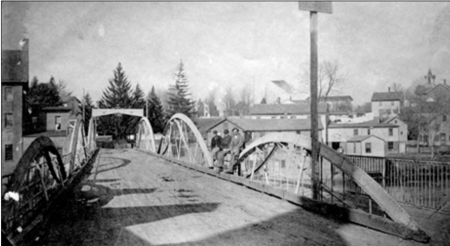
Early 1880s, looking northwest. In 1869, Moseley Iron Bridge & Roof Co., of Boston built an iron bridge to replace an old covered bridge that had been destroyed by fire. This bridge was, accordingly, referred to as the Moseley Bridge, as well as the Poquonock Bridge. WHS collections 1993.60.90B. Gift of William and Carrie Phelps Kendrick.
