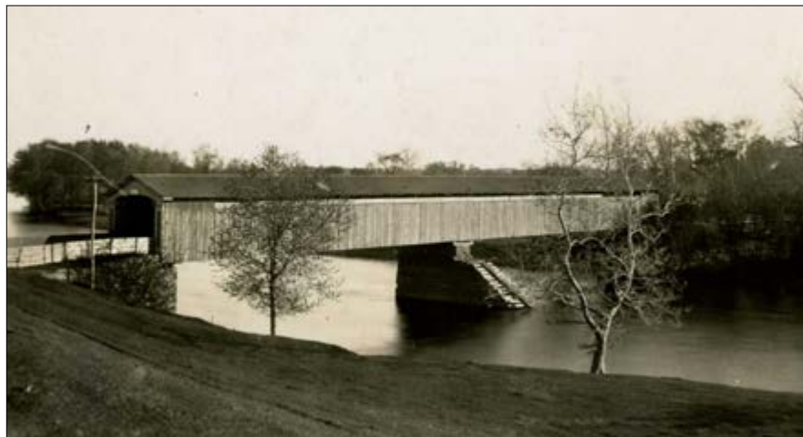
1860-1890s, looking southeast. This covered wooden truss bridge was built in 1854 and was sometimes called Fenton's Bridge. Alvin Fenton operated a general store out of his house, just up the street from here. The bridge's stepped center abutments were designed to break up ice floating downstream. WHS collections 2013.1.25.
