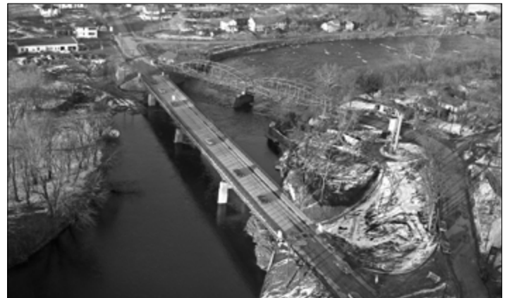
1953. After over a century of dangerous curves at the bottoms of hills on either end, the most recently built bridge finally straightened out Poquonock Ave. This photo shows the relationship between the old and new bridges, before the old was dismantled. WHS collections 2001.54.5. Photo by Philip Ellsworth Jr.
