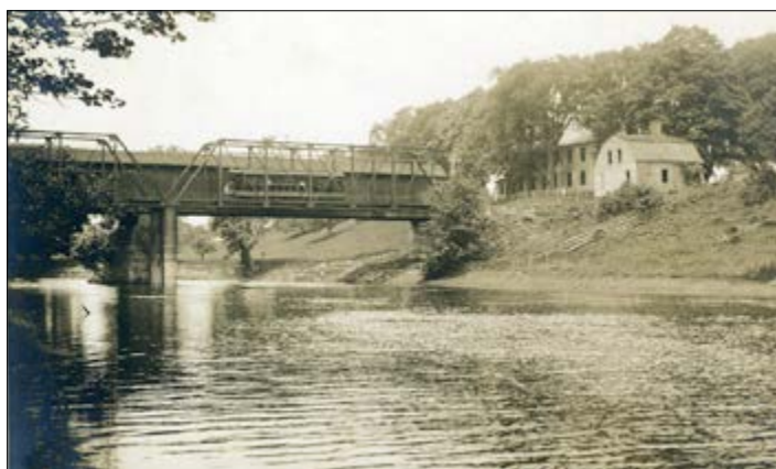
c.1904-1914, looking northeast. The trolley bridge on Palisado Ave. was built in 1904. This is the only photo we have of the "bridge house" that used to sit on the bank of the Farmington River. WHS collections 2014.42.81.
