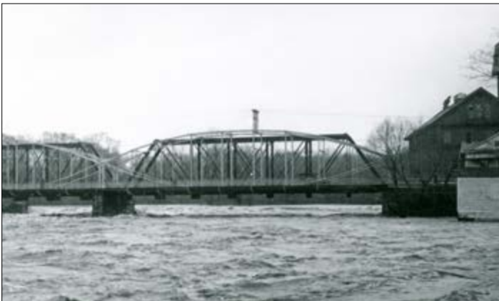
1936, looking west during the great flood. The trolley bridge was replaced around 1908. An enlarged Dunham Mill sits on the right. WHS collections 2000.30.183. Courtesy of Julius Rusavage.
